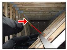
(2) Just past the note above. There is a two part truss system. The upper half of the truss is not seated fully. It is resting on the corner of the lower half and therefore the bottom of the top have has begun to split. Contact a licensed contractor for review and make repairs as needed.
