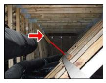
(2) Just past the note above. There is a two part truss system. The upper half of the truss is not seated fully. It is resting on the corner of the lower half and therefore the bottom of the top have has begun to split. Contact a licensed contractor for review and make repairs as needed.
