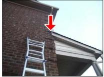
(2) All of the nails on the porch roof (and any on the upper roof) need to be removed to prevent them from landing in the gutter and or washing down the gutter into the yard to where someone could step on them.
