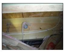
(2) Note: The band sill along the rear deck had no water damage or signs of wood destroying pest damage at the time of inspection.
