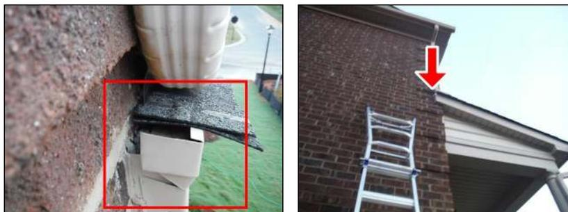
(2) All of the nails on the porch roof (and any on the upper roof) need to be removed to prevent them from landing in the gutter and or washing down the gutter into the yard to where someone could step on them.
