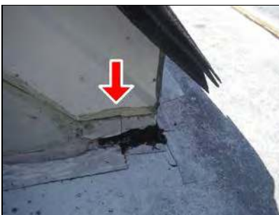
Tar tape flashing to fascia
