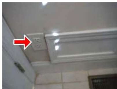
GFCI and access door
