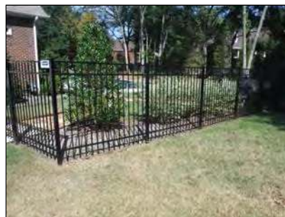
Installed pool and fence
