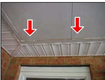
Tar tape flashing to fascia
