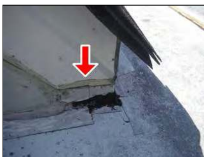
Tar tape flashing to fascia
